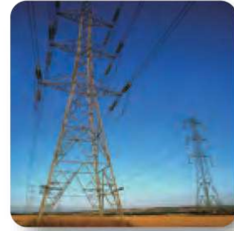
Electric Power Engineering
